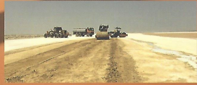
Polymer Road Construction Dammam KSA
